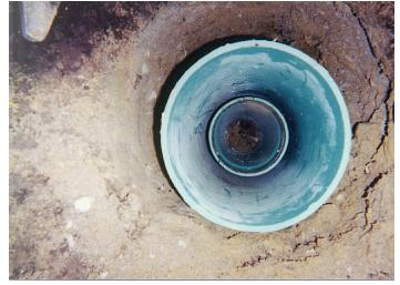
**Adding insulation and cabling** Add insulation to aid in thermal stability. Cut the 1" thick pipe insulation to fit the inside diameter of the 12" PVC pipe and line the PVC with the
