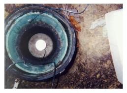
processor box. Feed the GPS, power, and data cable into the vault. leave a few extra feet on the cables length for convenience. Solder the connectors back onto the cables observing the exact wiring connection for each (the wiring diagram for each connection is in the PEPP manual).
